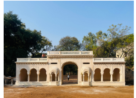
Rang Mahal after restoration
